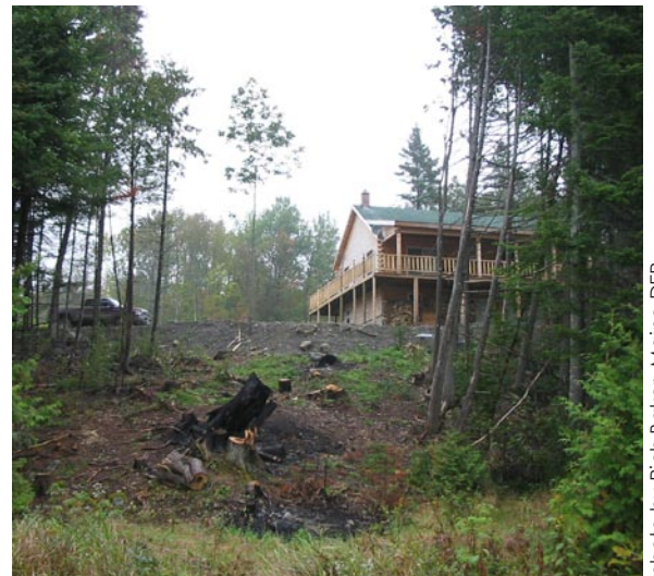
Cleared openings like this are prohibited within 100' of the shoreline through the MSZA.
