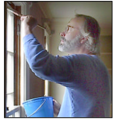
Paul Gregory paints windowsills in the living room
