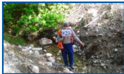
Severe erosion problems were identified and documented by volunteer surveyors.
